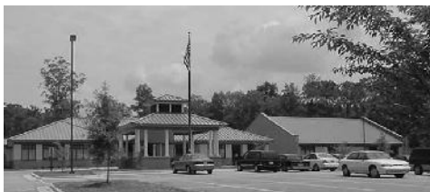
Cary Senior Center off High House Road inside of Fred G. Bond Park 120 Maury O'Dell Place
